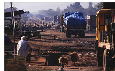
Figure 2. A roadway in poor condition in India.
